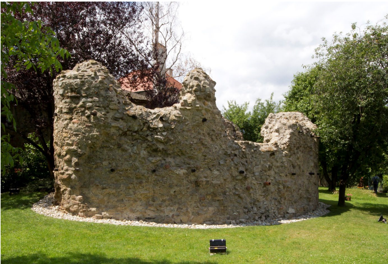
Zeiselmauer, fan-shaped tower (ID No 28d)
